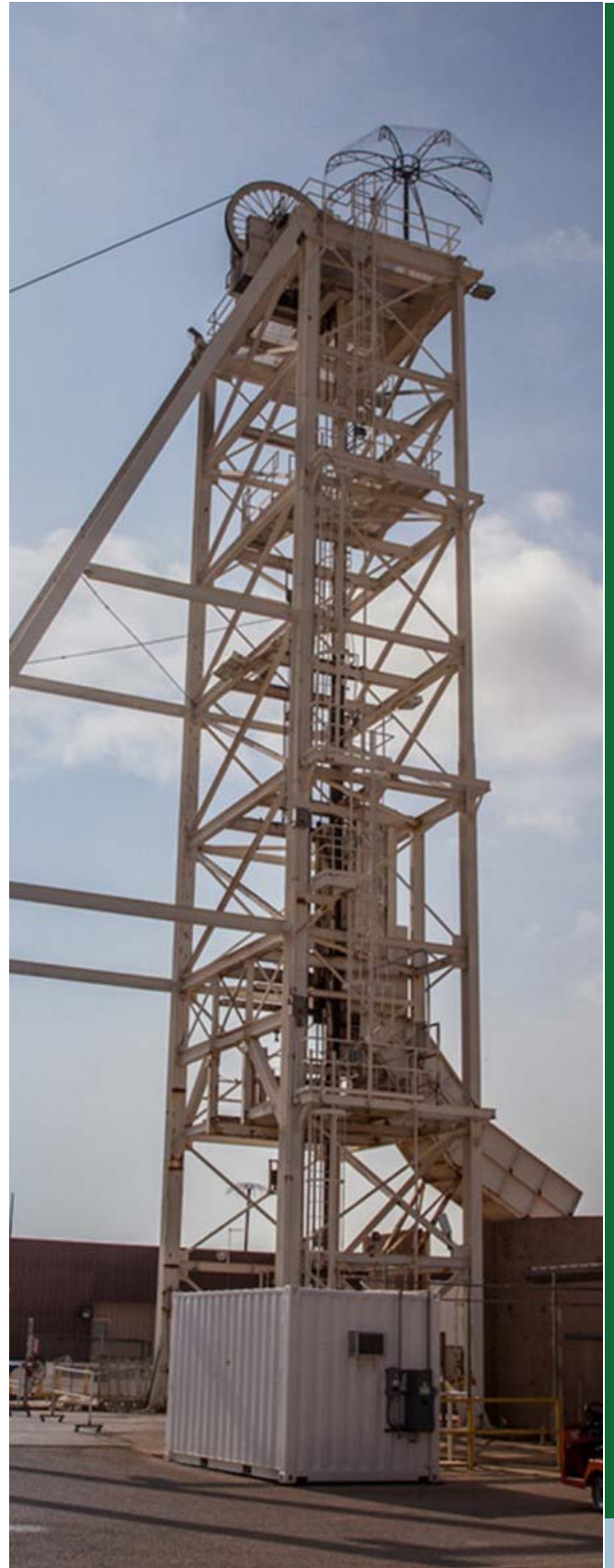
The Salt Hoist head-frame
