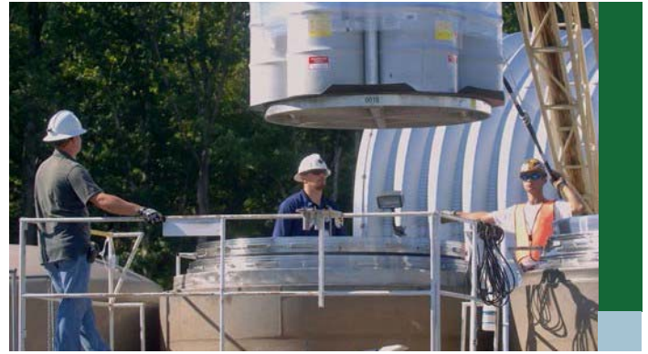
Mobile waste loading at a generator
